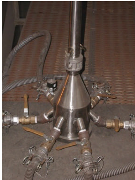
Figure 3. Distribution Manifold for Injection Lances at Plant Gaston
