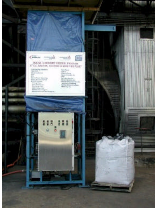
Figure 3. Distribution Manifold for Injection Lances at Plant Gaston
