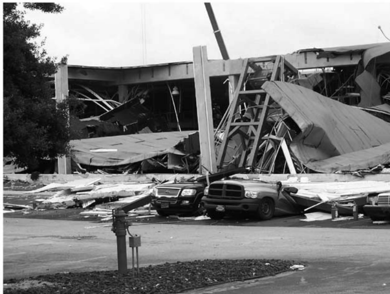
Figure 2. ConAgra Slim Jim meat processing plant in Garner, North Carolina, following the natural gas explosion of June 9, 2009, which killed 4 workers, injured 67 others, and caused much of the building to collapse.
