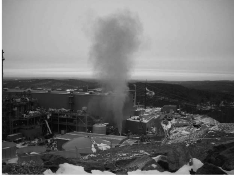
Figure 3. Natural gas blow conducted at the Kleen Energy plant a week prior to the explosion on February 7, 2010, showing plume of gas and debris hundreds of feet high.
