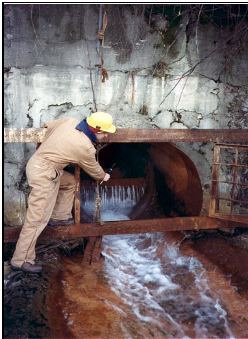
Figure 16 The Butler Mine Tunnel.
