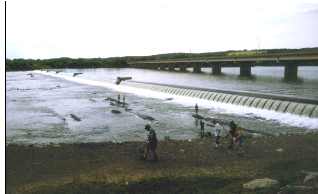
Figure 3 Sunbury inflatable dam inflated.
