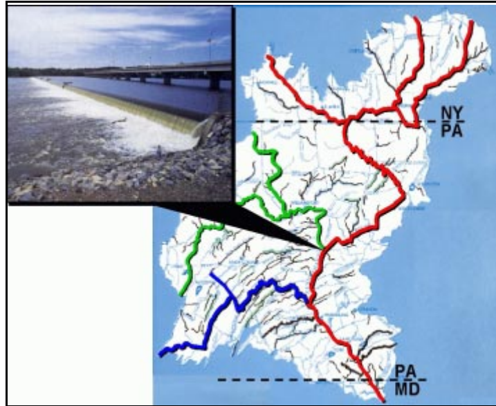
Figure 1 Inflatable Dam at Sunbury.
