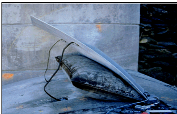
Figure 11 Side view of gate panel and bladder.
