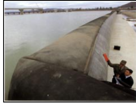
Figure 9 Inflatable dam at Sunbury.
