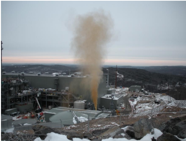
Figure 3. The cleaning of fuel gas piping at the Kleen Energy site on January 30, 2010, one week prior to the incident; a “gas blow” method was used to remove debris from the piping. The brown cloud seen here is indicative of debris being blown from the line.
