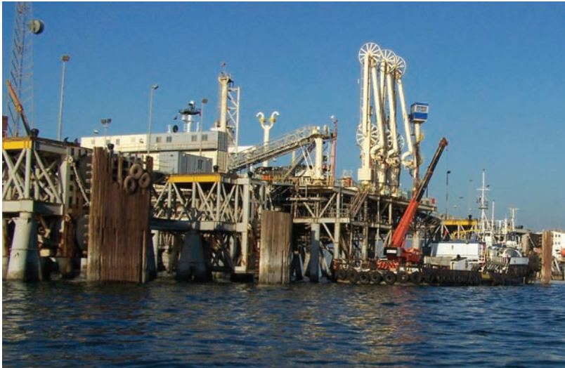
Loading arms at Al Basrah Oil Terminal.
