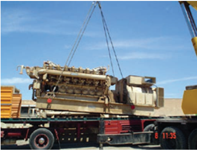
Cockrill generator removal. (Photo provided by USAID)
