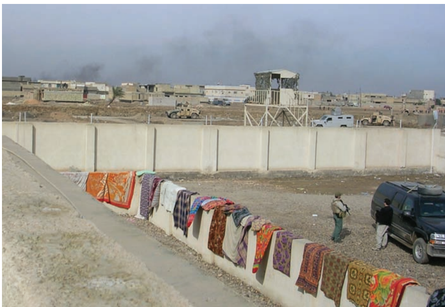
Security fence around police facility.
