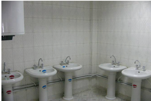
Barracks bathroom sinks and floor shortly after construction was completed. (Photo provided by Westin, Inc.)
