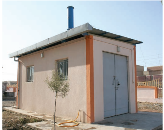
New incinerator was not used.
