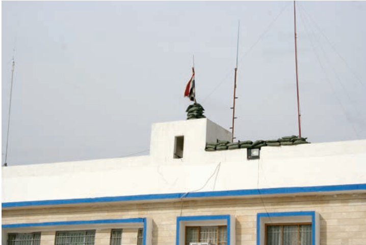
New rooftop guard houses and lighting upgrades improved force protection capability.
