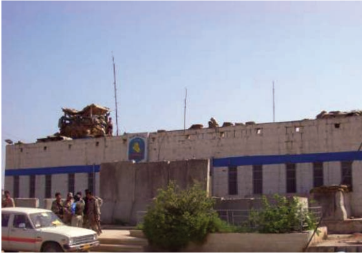
Site before construction: Inadequate guard houses, no security wall, open sewer culverts, and inadequate lighting.
