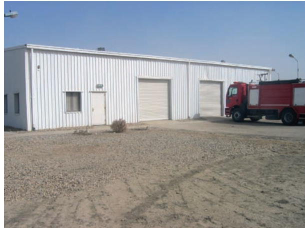
Tallil Military Base fire station.
