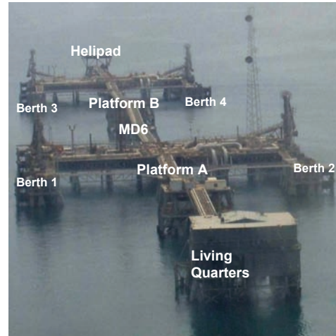
Aerial photo of ABOT platform. (Photo courtesy of USACE)
