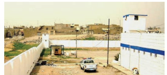
New guardhouse, new generator and fuel tank, new solid block wall and guard tower, and fresh paint.
