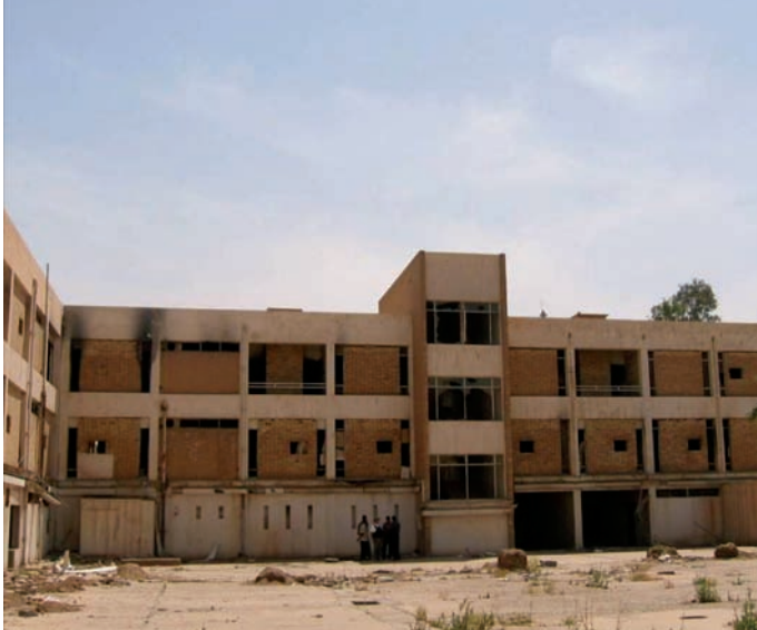
Exterior view of ICD HQ prior to renovation.
