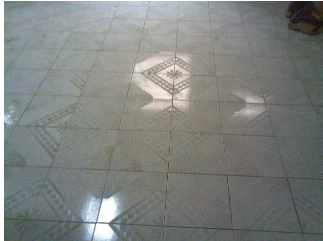
Bathroom floor repair by contractor after SIGIR's inspection. (Photo provided by Westin, Inc.)
