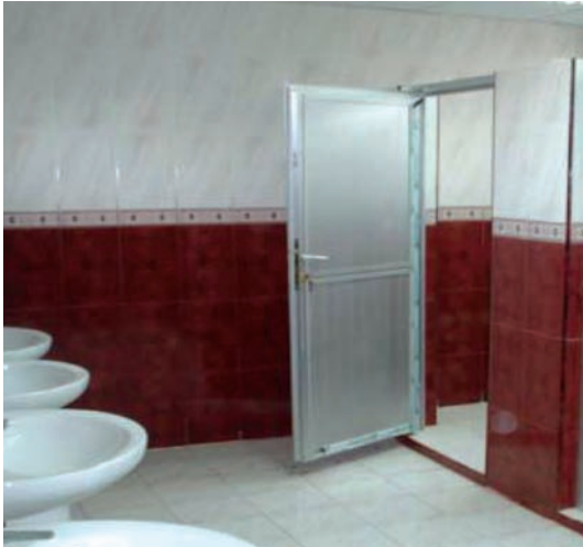
External toilet following renovation. (USACE photo, January 18, 2006)
