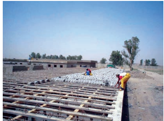
"Omni" blocks were placed on evenly spaced concrete beams.
