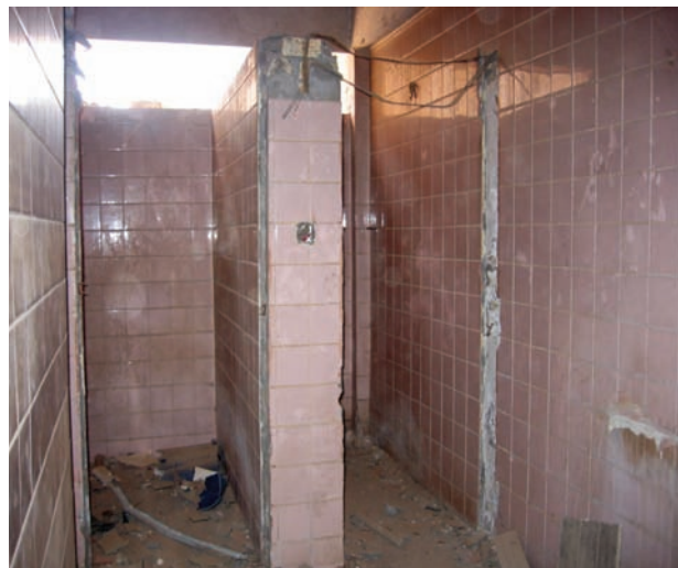
Condition of bathroom prior to renovation.
