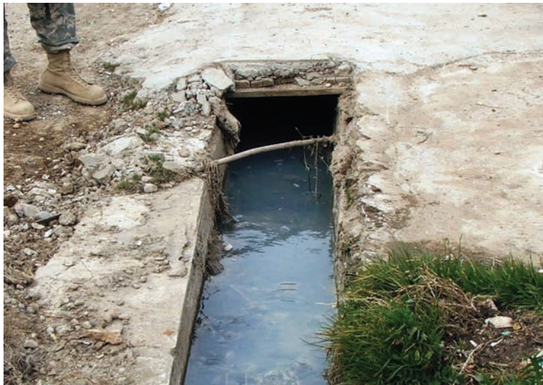
Concrete over sewer culvert was cast too thin, cast without rebar or reinforcement wire and not uniformly mixed.
