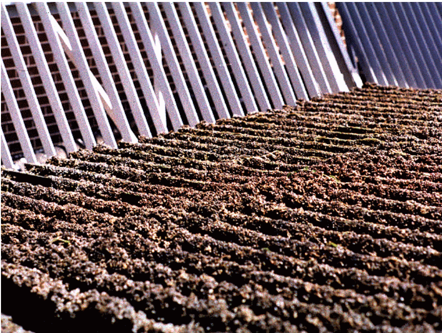
Figure 2 – Zebra mussel fouled trash rack
