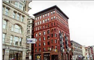
Scranton's Historic District, courtesy of National Park Service
