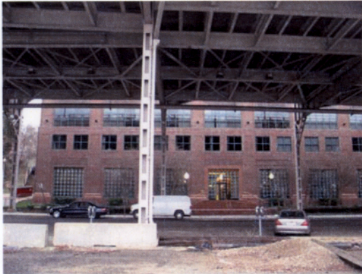
Front view showing freeway
