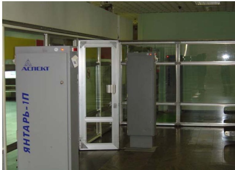
Figure 8. RPMs in Russia to screen air passengers and baggage.
