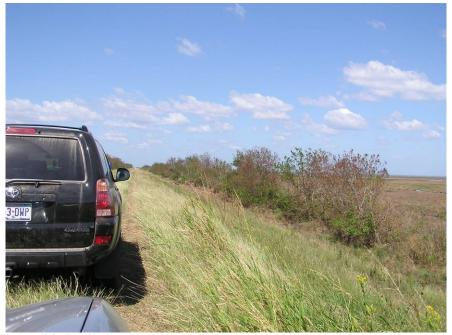
Figure 3.16: Virtually unscathed earth embankment levee on the eastern edge of the protected area of New Orleans East
