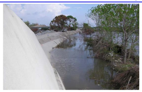
Figure 2.17: The toppled floodwall/sheetpile walls at the London Avenue Canal (North) breach site.
