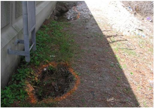
Figure 2.21: Closeup view of sinkholes at the inboard toe of the floodwall, at the location of the engineer wearing a red shirt in Figure 2.20.
