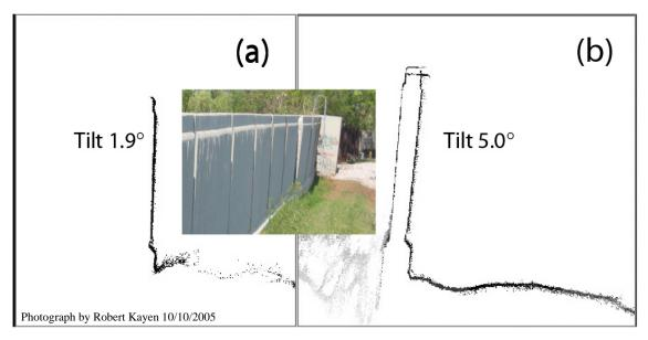
Figure 7.14: Cross sections through two segments of distressed I-wall at London Avenue Canal. Segment (a) is toward the south (left) of Figure 7.13 and has a modest 1.9 degree rotational deformation toward the landside of the levee. Near a position of maximum distress, the I-wall has 5.0 degrees of rotational deformation.
