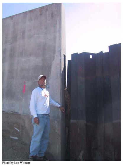
Figure 3.19: Transition between concrete and sheetpile walls at uneven wall height elevations
