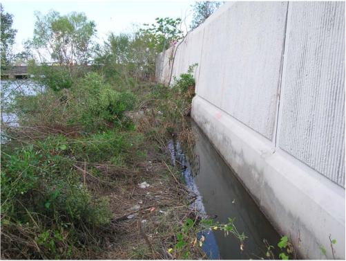
Figure 2.19: Gap at the base of the floodwall on the canal side of the East Bank "distressed" section.
