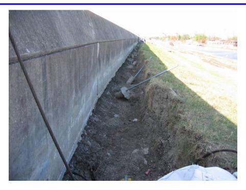
Figure 4.4: North view from the end of the south breach of Lower Ninth Ward. Note how the scour trench becomes progressively wider as it approaches the breach (J. Wartman, October 4, 2005).
