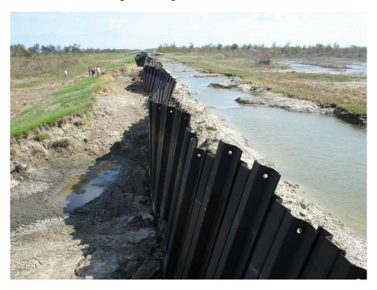
Figure 4.20: Failure of earth levee with steel sheetpile barrier on the southeast bank of the MRGO. Note severe erosion and scour (L. Wooten, October 6, 2005).
