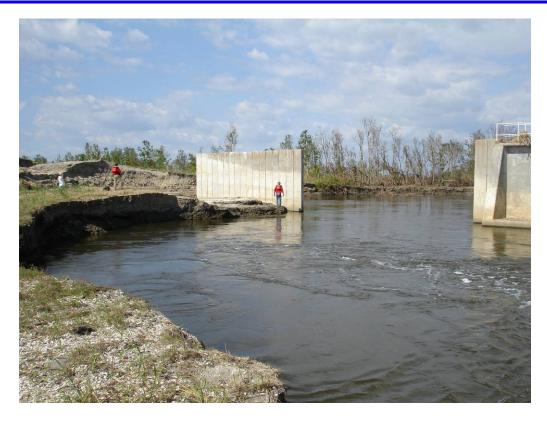
Figure 4.23: Ground perspective of Bayou Dupree gate abutment failure (L. Wooten, October 6, 2005).
