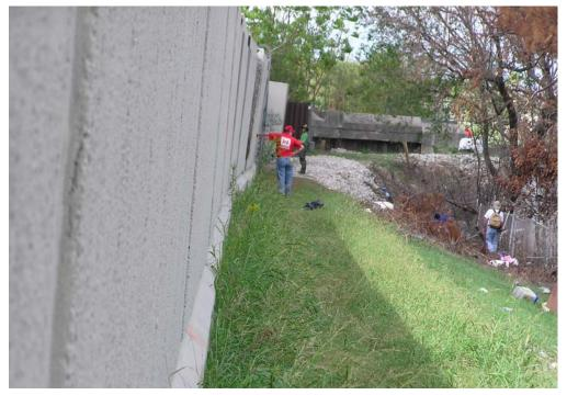
Figure 2.20: View of the inboard side of the floodwall and earthen levee embankment.
