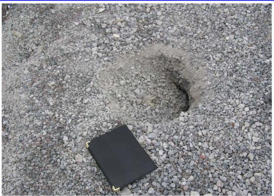
Figure 2.13: One of four sinkholes noted at the front lip of the crest of the temporary closure section embankment.
