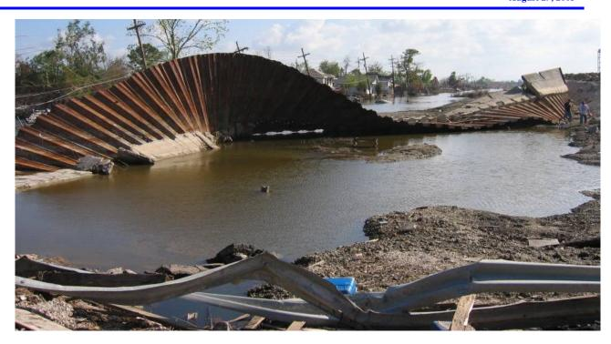
Figure 4.10: Overturned I-wall system at north breach of Lower Ninth Ward (J. Wartman, October 4, 2005).
