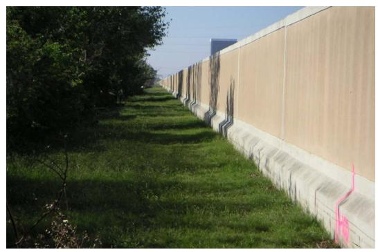
Figure 2.11: Typical conditions at the inboard side of floodwalls along the 17<sup>th</sup> Street Canal showing no scour of soil at the toe of the wall.
