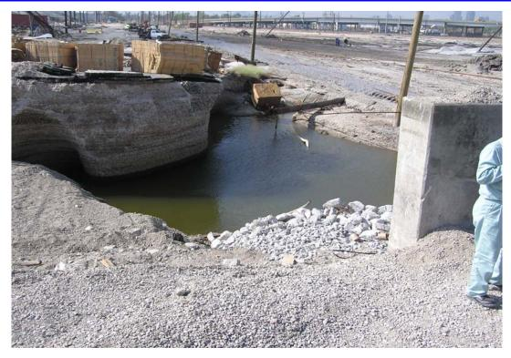
Figure 2.29: Erosion at a "transition" between a concrete floodgate wall and the adjacent earthen embankment section.
