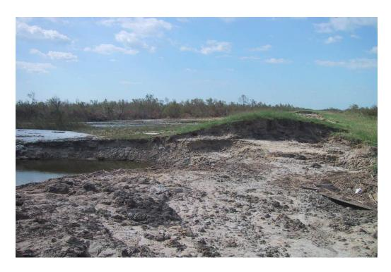
Figure 4.24: Failure of earth levee on southwest bank of MRGO adjacent to the Bayou Dupree gate (L. Wooten, October 6, 2005).
