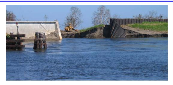
Figure 4.13: Sheet pile breach at the Bayou Bienvenue Gate (J. Wartman, October 5, 2005).
