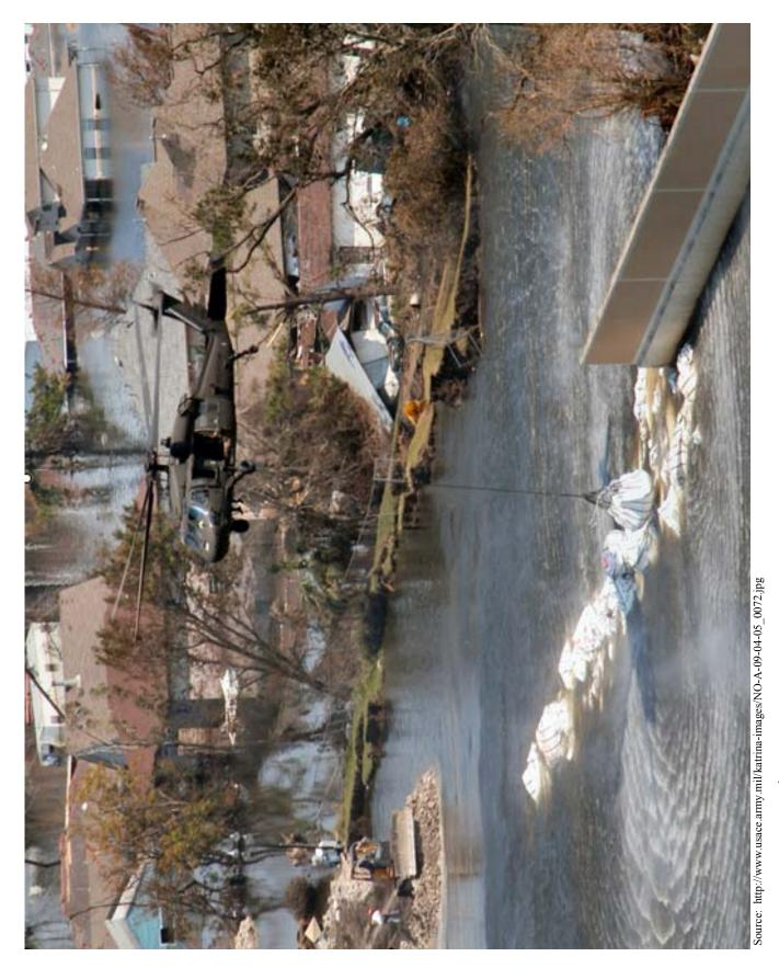
Figure 2.3(a): The 17<sup>th</sup> Street Canal breach during initial breach closure.
