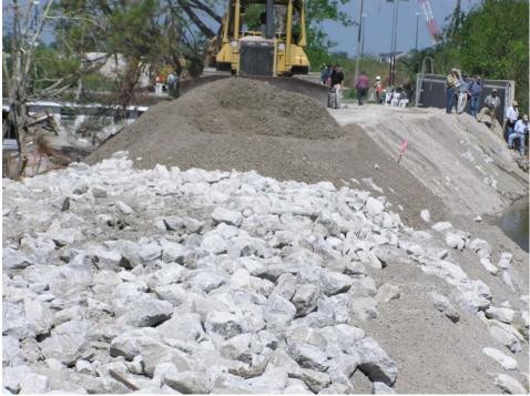
Figure 2.23: Photo during construction of the emergency breach repair embankment at the London Avenue Canal (North) breach site.
