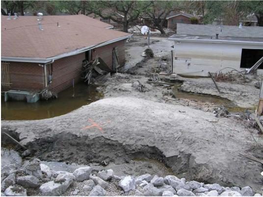
Figure 2.18: Sediment from the London Avenue Canal was deposited inboard of the levee break. High water marks (from long-term ponding) are visible on the exteriors of the residential homes.
