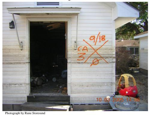
Figure 1.8: High water marks remain on structures after temporary levee repairs have been completed and flood waters have been pumped out.
