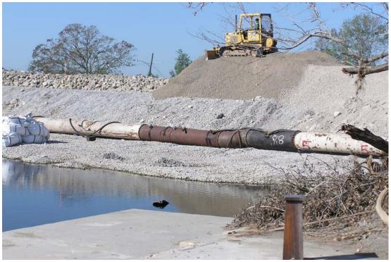
Figure 2.14: Placement of silty sand fill at the crest and on both the inboard and outboard faces of the temporary embankment closure section on October 6, 2005.
