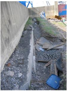
Figure 4.8: A scoured, but nevertheless well-performing "T-wall" levee section located near the north breach of the Lower Ninth Ward (J. Wartman, October 4, 2005).
