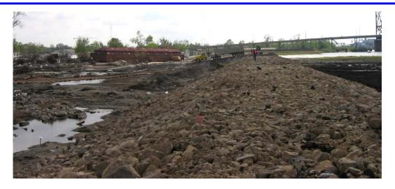
Figure 4.6: South view of the south breach repair at the Lower Ninth Ward (J. Wartman, October 4, 2005).
