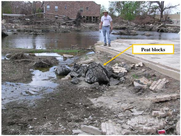
Figure 2.5: View from crest of emergency embankment closure section at the 17<sup>th</sup> Street Canal breach, looking south across the floodwater scoured zone.
