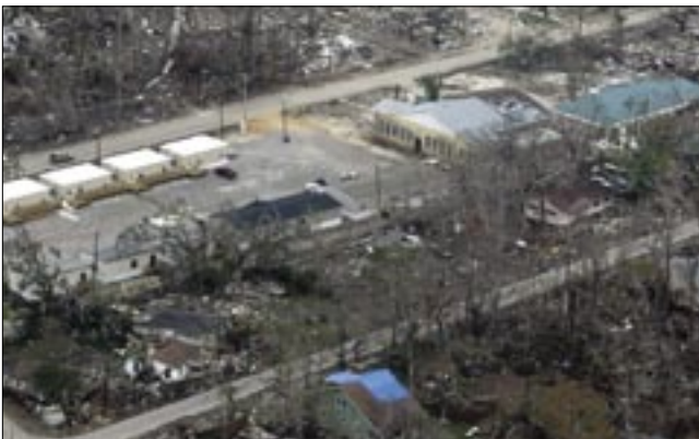
FEMA-provided temporary buildings out of which Waveland's city government, including its police department, is now operating.
