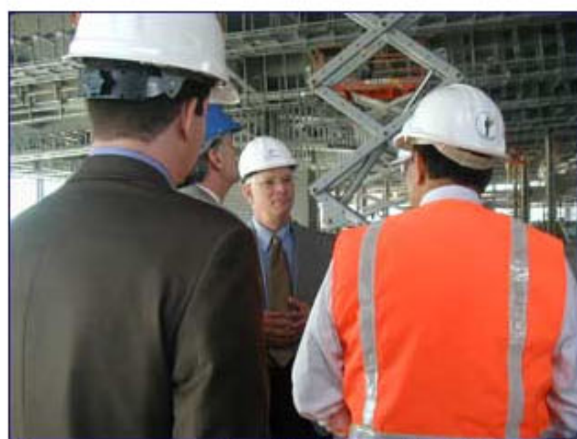
Congressman Cardin Tours BWI Airport Construction Site
